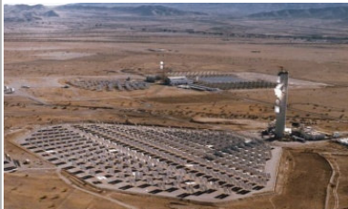
Solarised gas turbines
